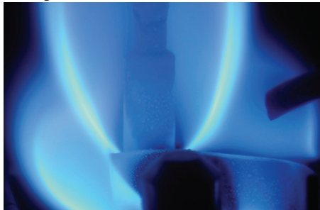
Blue flames can indicate efficient burner operation.
