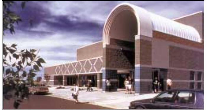
Oñate High School in Las Cruces, New Mexico, incorporates individual heat pumps for each classroom.
